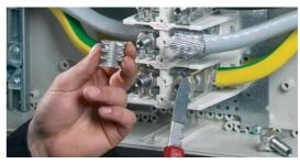
4. The steps listed above need to be repeated if the conductor is removed and re-connected. I.e. the conductor has to be scraped again, greased and immediately connected, because it will be connected at a different position.
