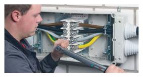
3. Due to the flow tendency in aluminum the terminals need to be tightened before start up and after the first 200 operating hours (note the appropriate torque).
