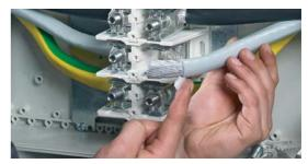
2. Immediately after removing the oxide layer, the conductor end needs to be rubbed with an acid and alkali free grease such as technical vaseline and then immediately connected to the terminal. This in turn prevents oxygen from forming a nonconducting oxide layer.
