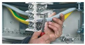
1. The non-insulated conductor ends need to have the oxide layer carefully scraped clean using a knife for example. In doing so no files, sand paper or brushes may be used.
